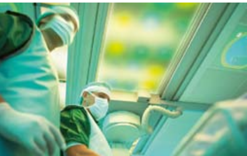
A 'skylight' provides thematic lighting for the patient and procedural lighting for the staff
